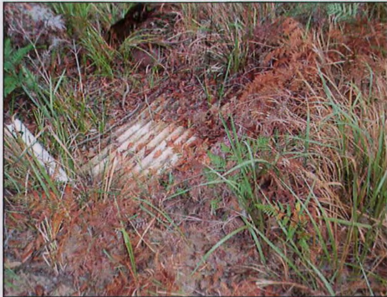
Photo 1. Panels of corrugated FCS in north eastern part of the site.
